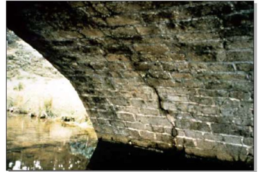
Longitudinal crack inside the vault
