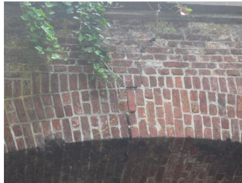
Transversal crack at the top of the vault
