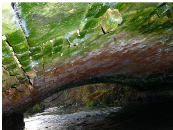
Defective jointing Poor waterproofing Stone removal
