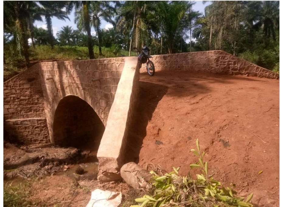
Backfill Deck Kilema Bridge Mkongoro - Kigoma
