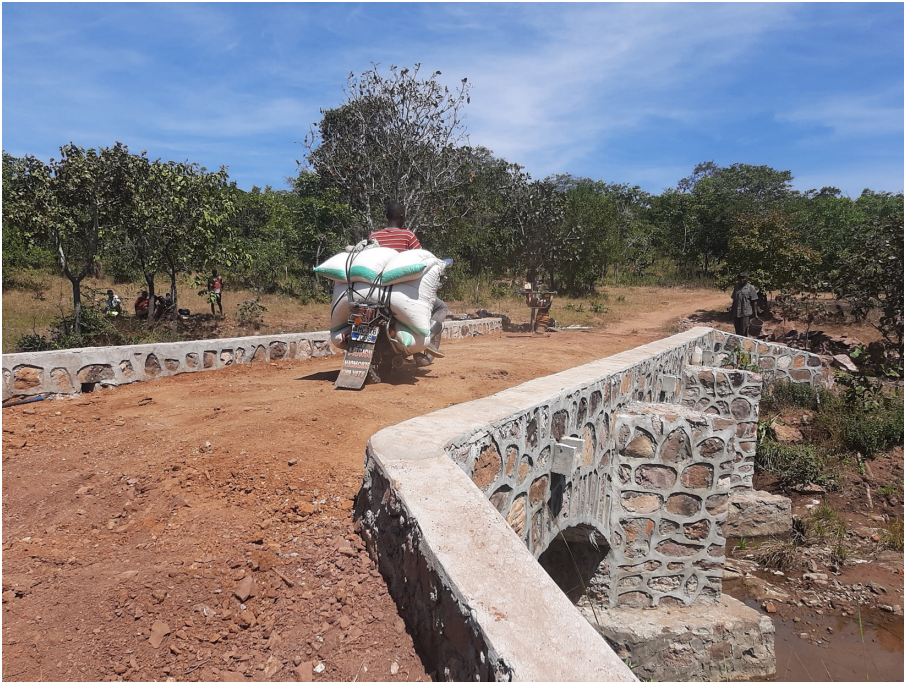
Backfill Deck Kacheli Bridge Uvinza - Kigoma
