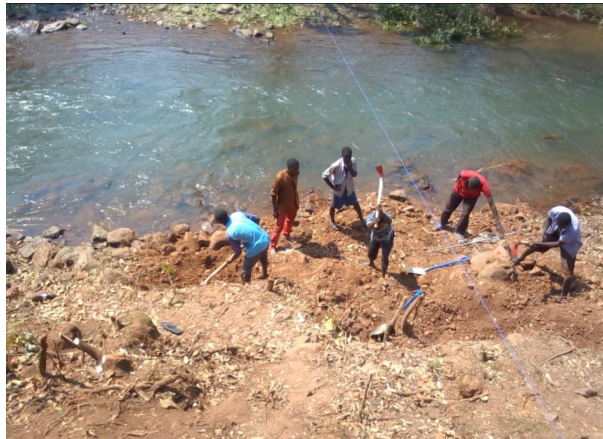
Initial Excavation via Labour based technology by the Villagers
